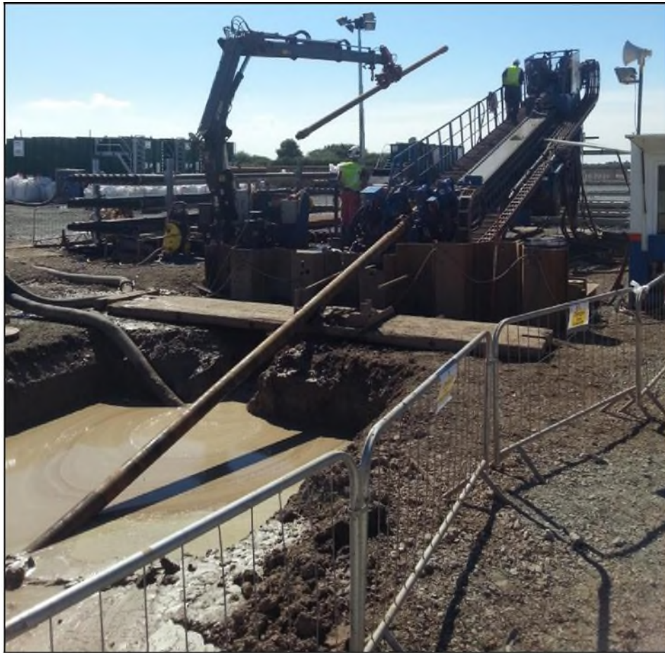
Figure 4.18: HDD rig carrying out landfall works at the Westermost Rough offshore wind farm
